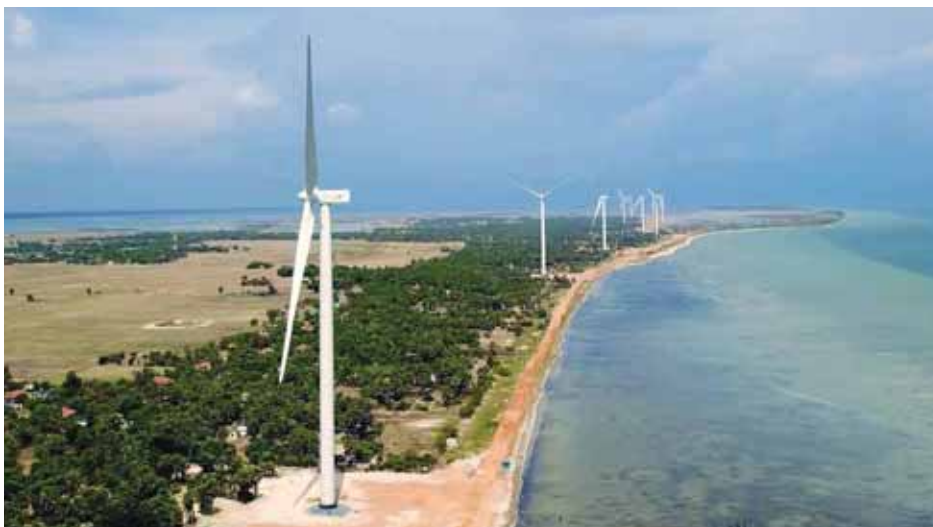
Two wind power projects (10 Mw each) in Jaffna peninsula funded by NDB PIF, started their successful commercial operations in 2020
