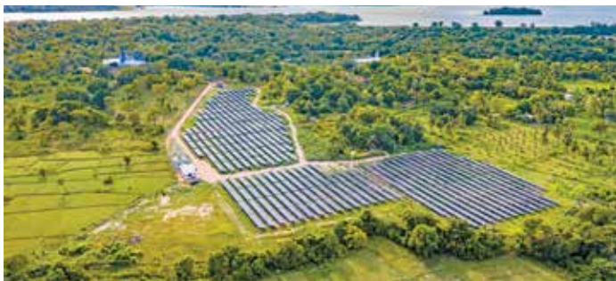
Ground mounted solar projects in Nachchaduwa, Anuradhapura
